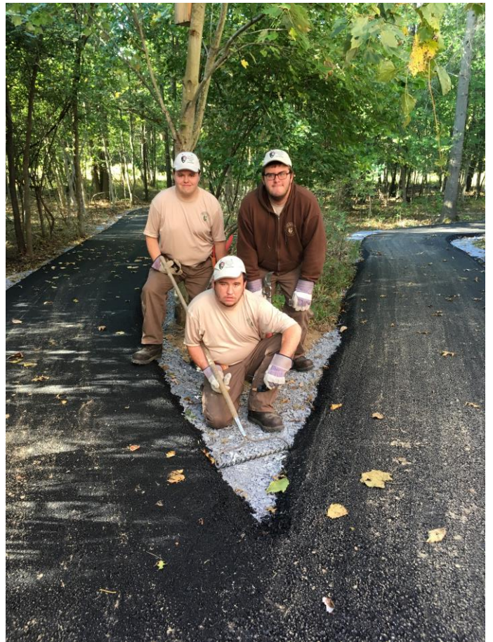
Crew rests after stone base and blacktop finished
