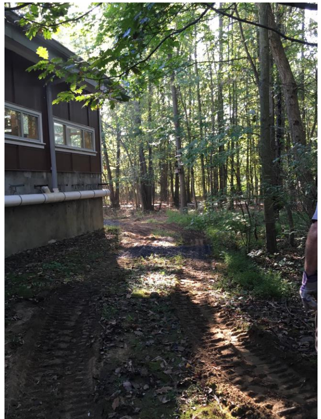
Part of trail before stone base is laid
