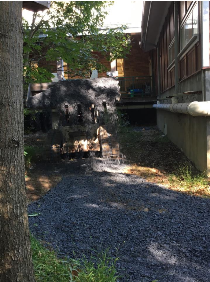
Laying the stone base
