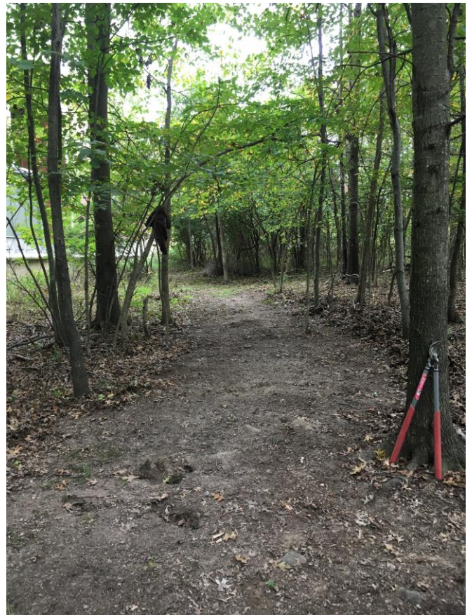
Trail cleared and ready for base stone
