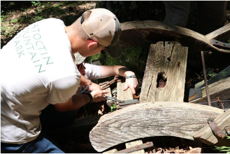
Disassembling the historic charcoal shed
