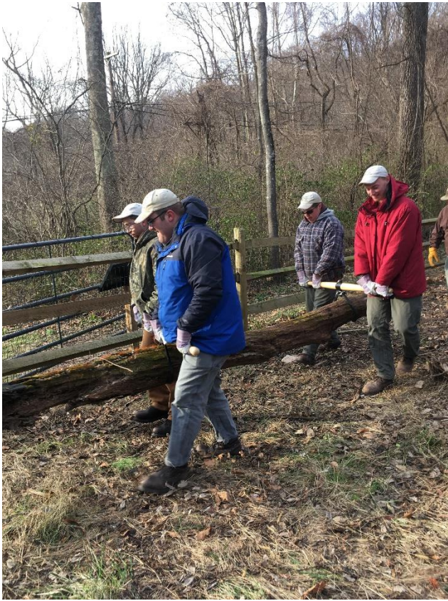
Moving a log with a log carrier at the Ironmaster's House at Catoclin Furnace
