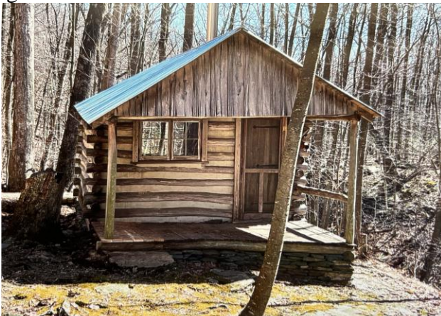
New tin roof on cabin at ThorpeWood
