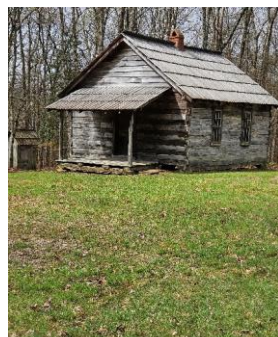
School House with outhouse to left (roof repair)
