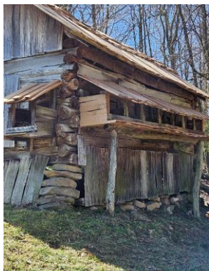
Henhouse boxes and roof repaired
