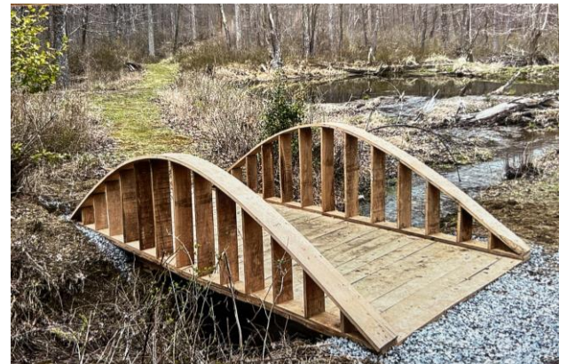
New bridge at ThorpeWood. Notice the bent wood railing.
